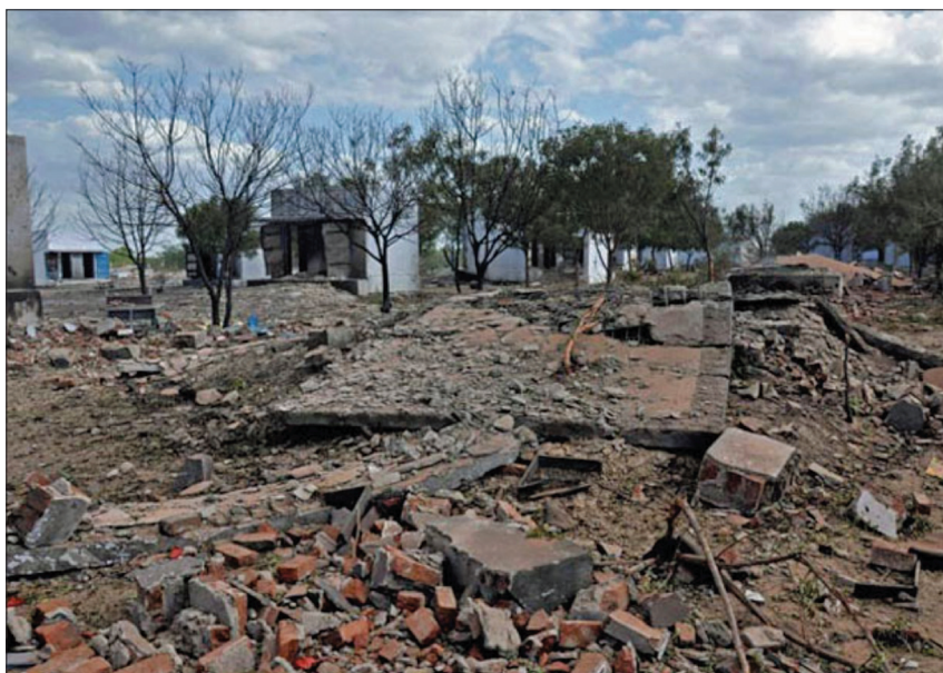
Figure 5.5: Site of Om Shakti Fireworks after explosion
