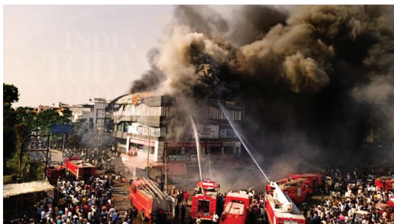
Figure 8.3: Fire at Takshashila Arcade on May 24, 2019
