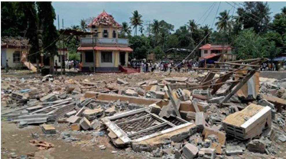
Figure 7.3: The destroyed temple complex after the explosion
