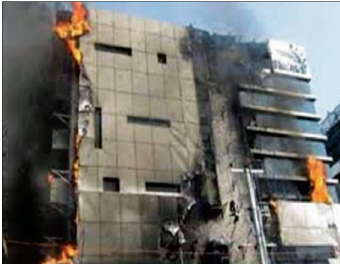
Figure 4.3: The fire reached to the top floors of the AMRI Hospital
