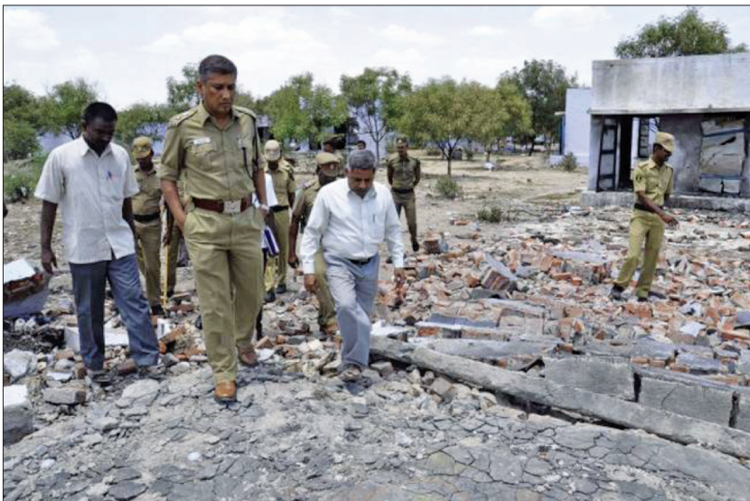
Figure 5.6: Najmul Hoda, Superintendent of Police, Virudhunagar inspecting the flattened shed where the fire had allegedly originated.
