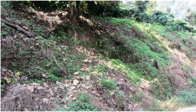
Photo:1 Slope failure (Chittalli-Madikere road)
