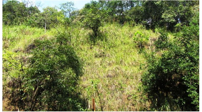
Photo:2 Old slide scar (Perumbadi-makutta road)
