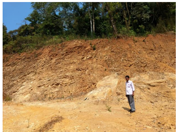
Photo:22 SFM class weathered rock, T.S No. 48P/11, near Korangala village.
