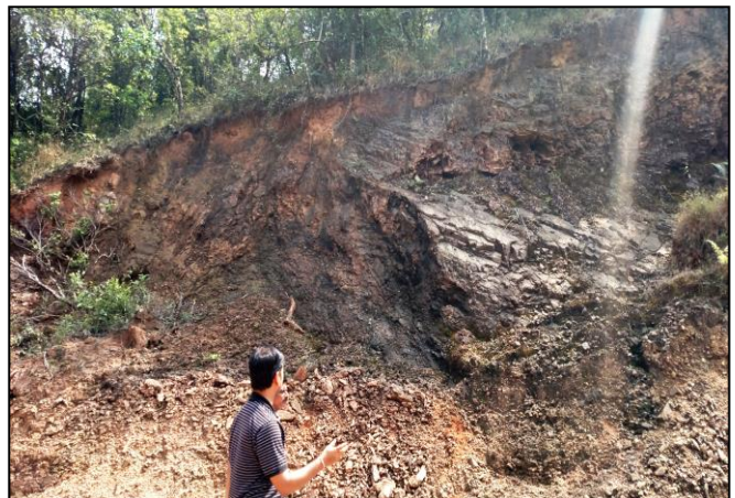
Photo: 4 Debris slide on Talakaveri – Korangla road, T.S. No. 48P/11.
