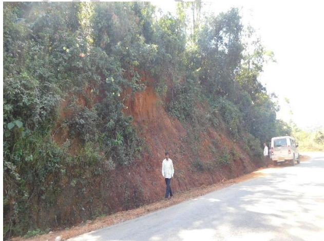
Photo 4.1c Extensive slope cut (Lat: 13°50'55.98" Long: 75° 03'50.04")
