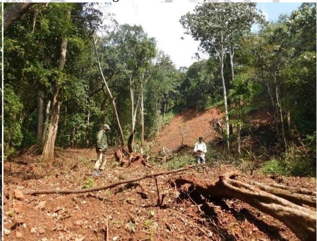
Photo 3. 1d Debris flow near Hanigeri village Lat: 13°51' 58.88" Long: 75° 25' 8.30")
