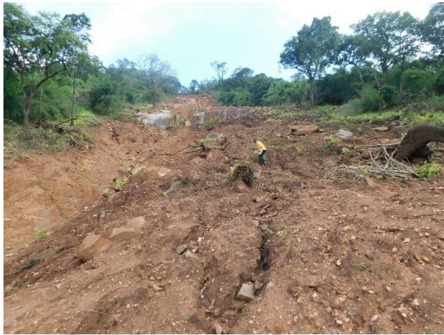
Photo 3. 1a Debris flow near Hegalathi village (Lat:13° 50'7.27" Long: 74° 27'1 49.20")
