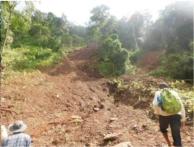
Photo 3. 1b Debris flow near Hanigeri village (Lat: 13° 51' 13.71" Long: 75° 25' 21.87")
