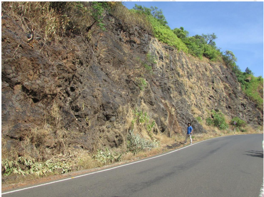
Fig. 4.5: Extensive Slope Cut along Keri – Chorla road near Chorla.
