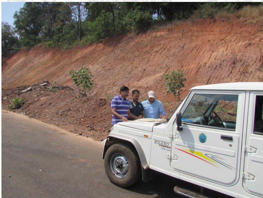
Fig. 4.20: In-situ soil present as slope forming material near Ponda.
