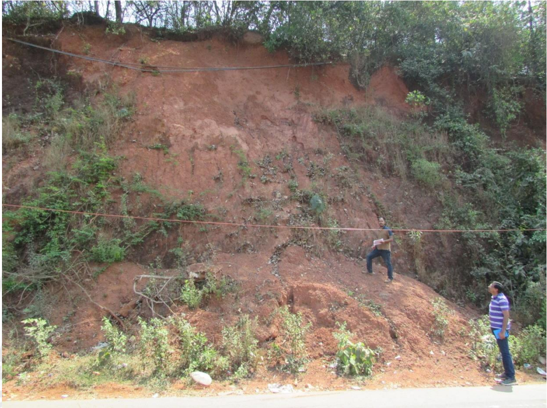
Fig. 3.9: Active debris slide along Borim - Ponda bypass road (slide Name: GOA/SG/48I03/2020/23).
