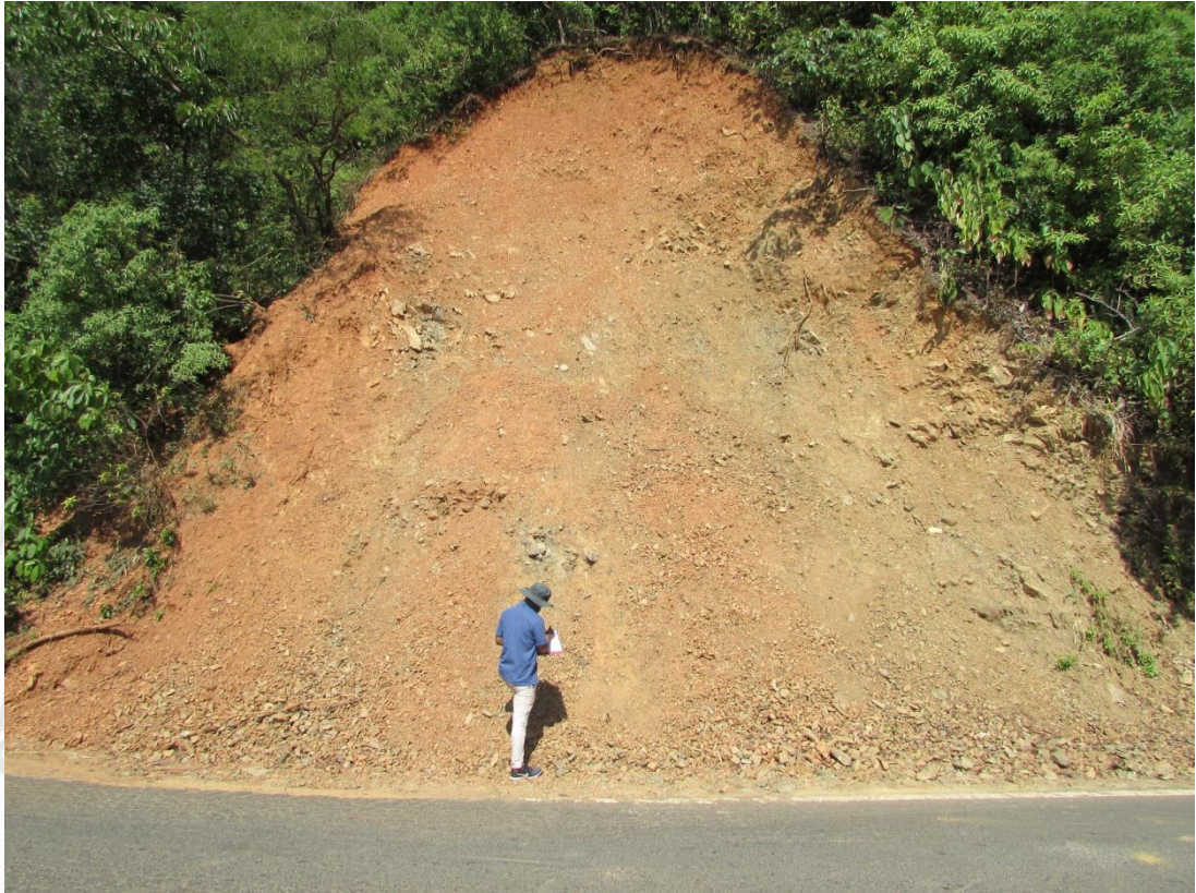
Fig. 3.5: Active debris slide along Chorla Ghat road (slide Name: GOA/NG/48I02/2019/15).
