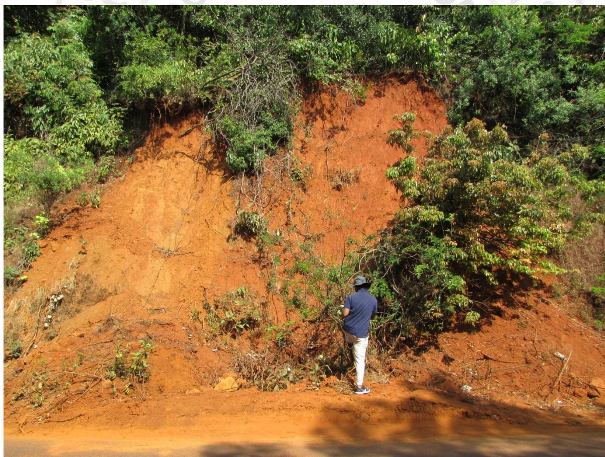
Field photograph of landslide no: KAR/BEL/48I02/2019/20
