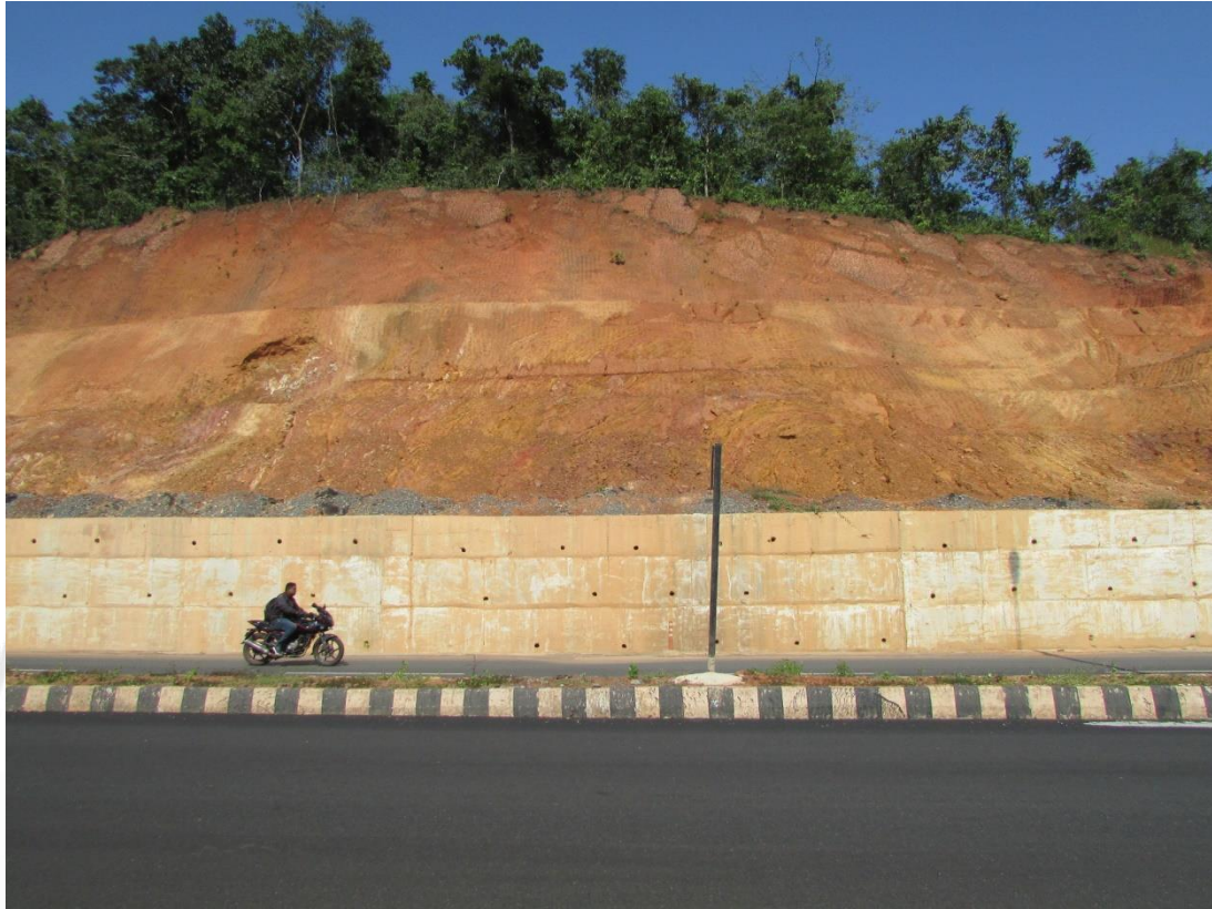
Fig. 4.25: Regolith Thickness >10 m near Ponda.
