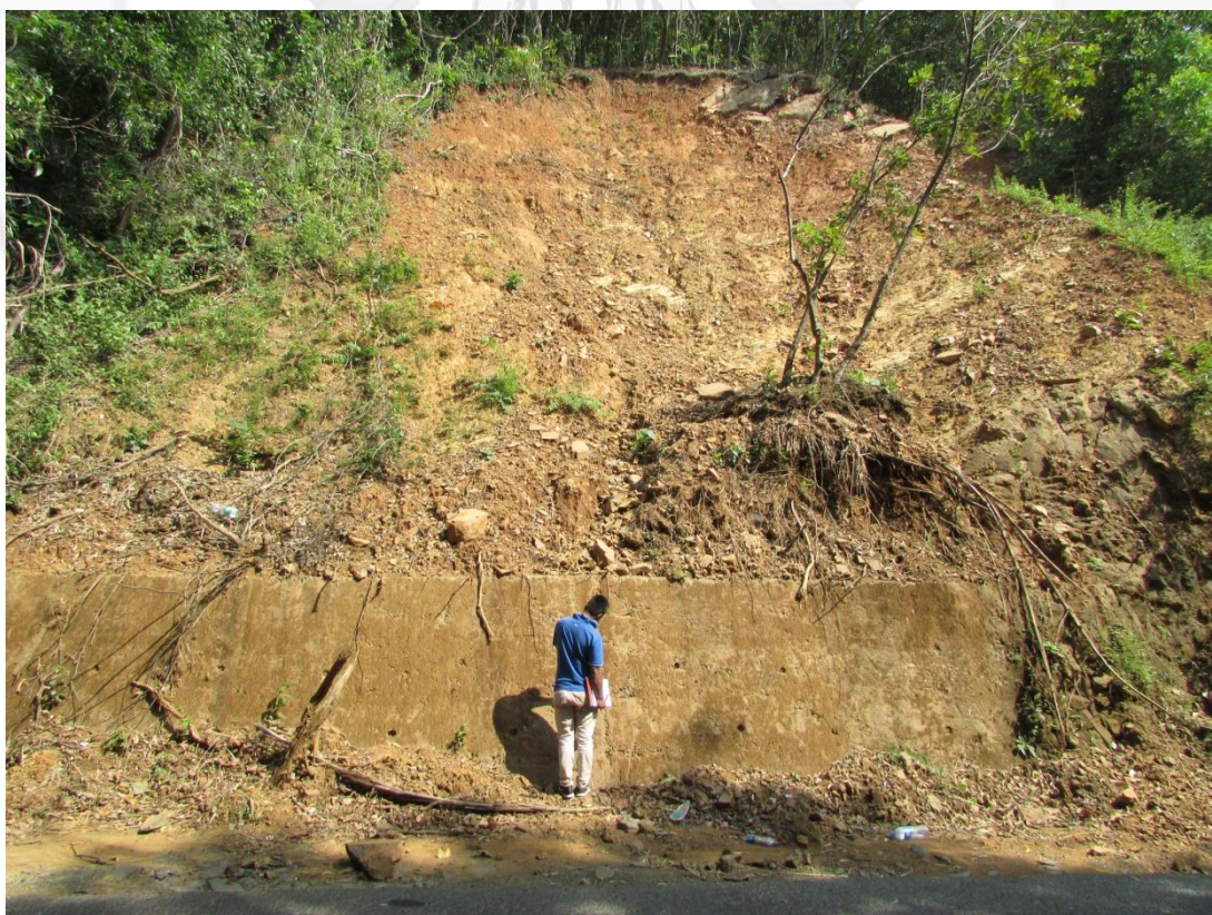
Fig. 3.4: Reactivated debris slide along Chorla Ghat road (slide Name: GOA/NG/48I02/2019/13).
