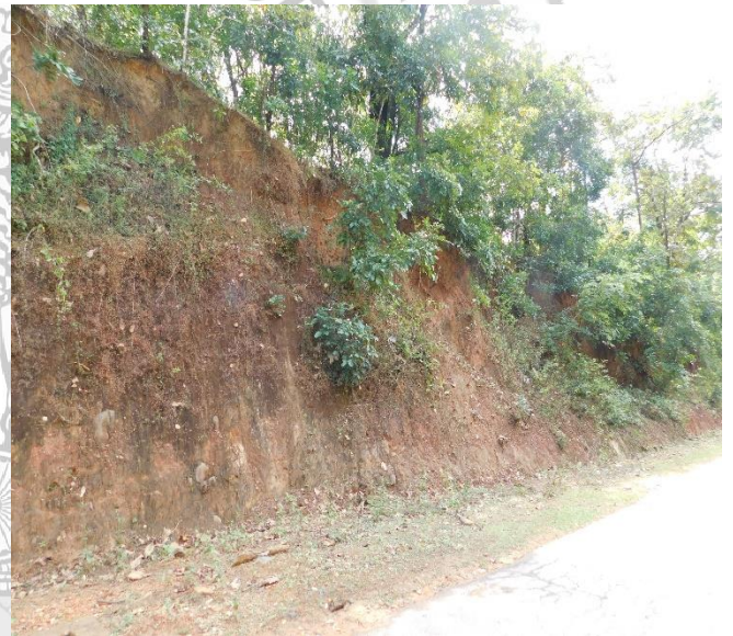
Photo- 22: ECS on Vartigundi-Dupadakan road section
