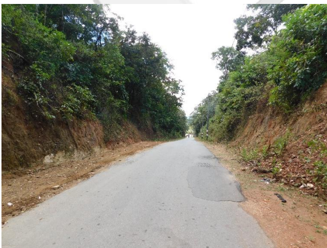
Photo- 23: ECS on Guladamane-NR Pura road section
