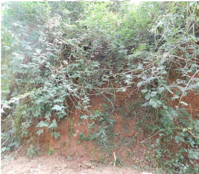
Photo- 21: ECS on Santaveri-Chikmagalur road section
