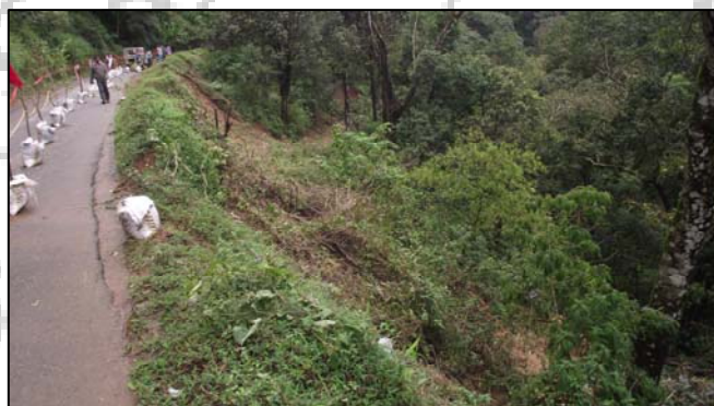
Photo 24: View of landslide near Kattalekadu on SH-89 between Madikeri-Chettali.
