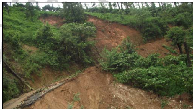
Photo 14: View of first Landslide on Makandur-Mukkodlu tantipal road.
