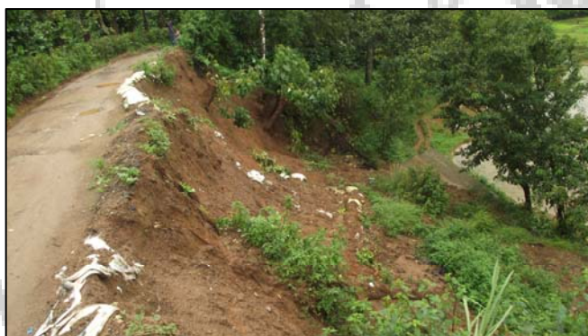
Photo 17: View of landslide near Makandur village, Sinchona estate road.
