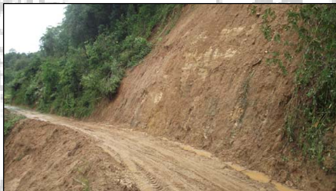
Photo 16: View of the Hattihole-Avandi road landslide with fresh gneissic bed rock exposed.
