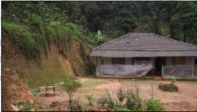
Photo 3: House of Shri. Jayaprakash in Mannangeri village constructed on nala course by slope cutting
