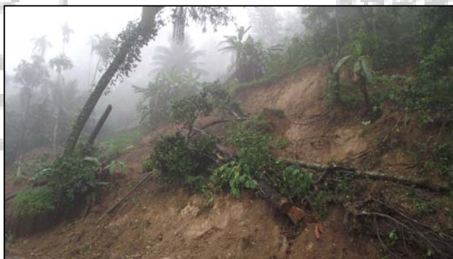
Photo 27: View of landslide near Jodpal on SH-88 between Madikeri-Sampaje.
