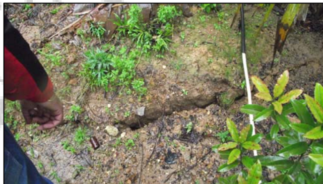
Photo 8: Cracks seen besides house of Smt. Sitamma in Makandur village.
